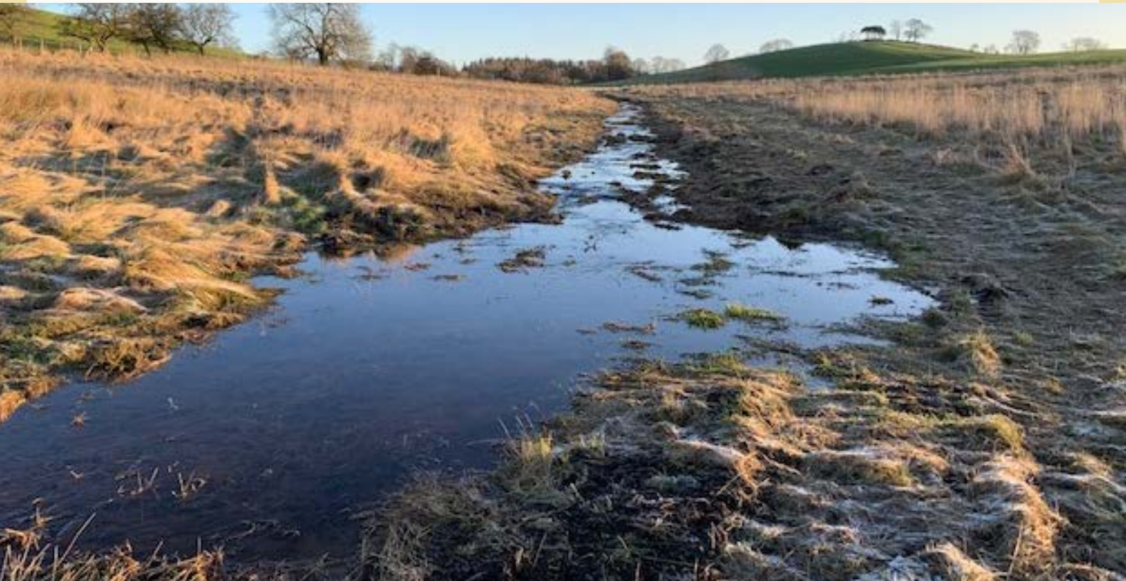
Deculverting at Skinner Ground, January 2022
